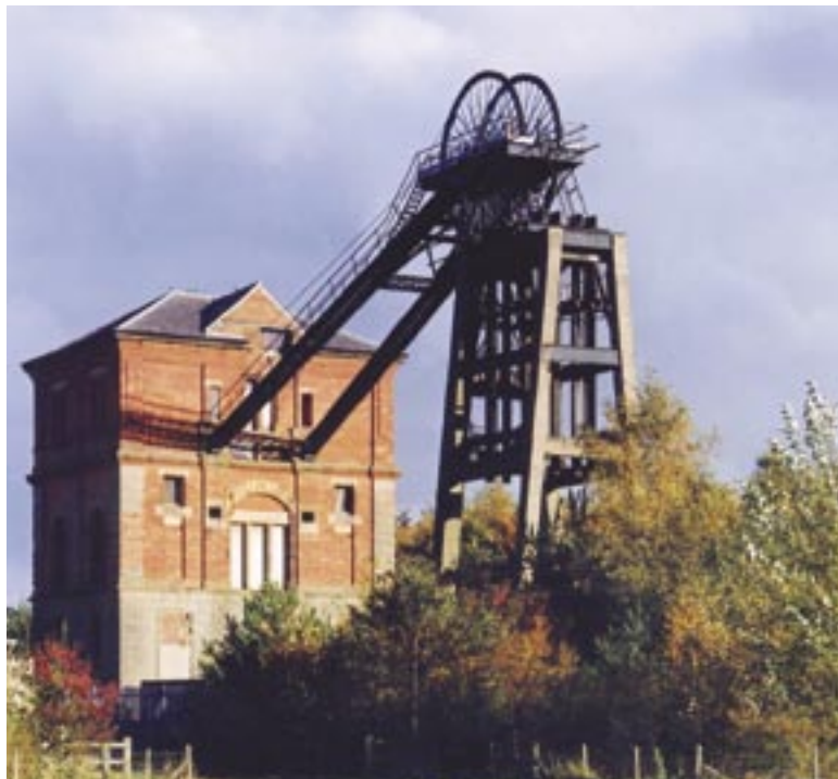
Bestwood Winding Engine House
